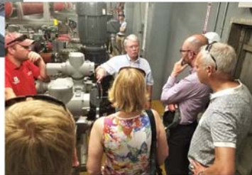
Left—I-Storm members with Steve Spencer at the Surge Barrier Sector Gate
